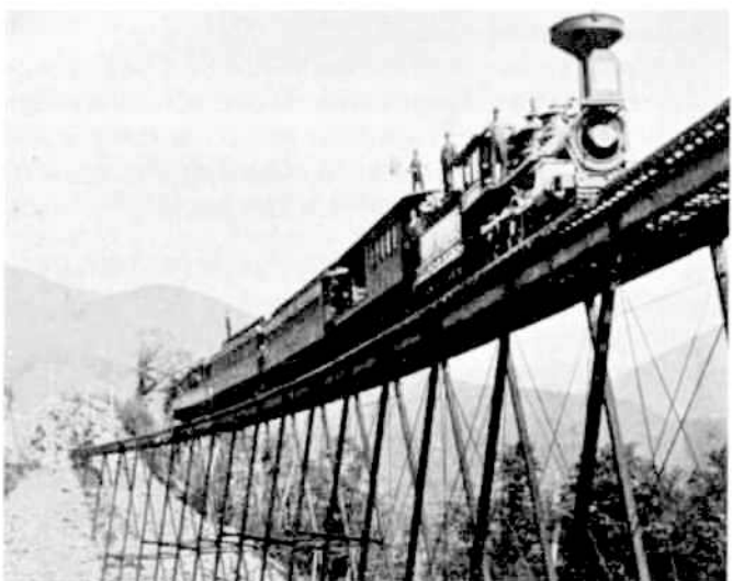
Frankenstein Trestle, P. & O.R.R., Crawford Notch
