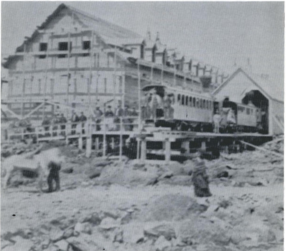
New Summit House under construction, 1873.
